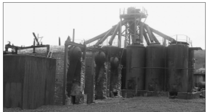
Boilers and blubber digesters are exposed to the public gaze.
