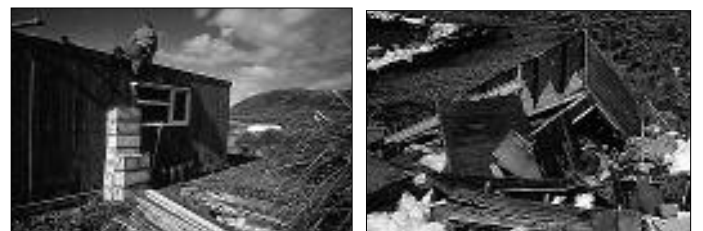
Arnov House: before and after the wave.
