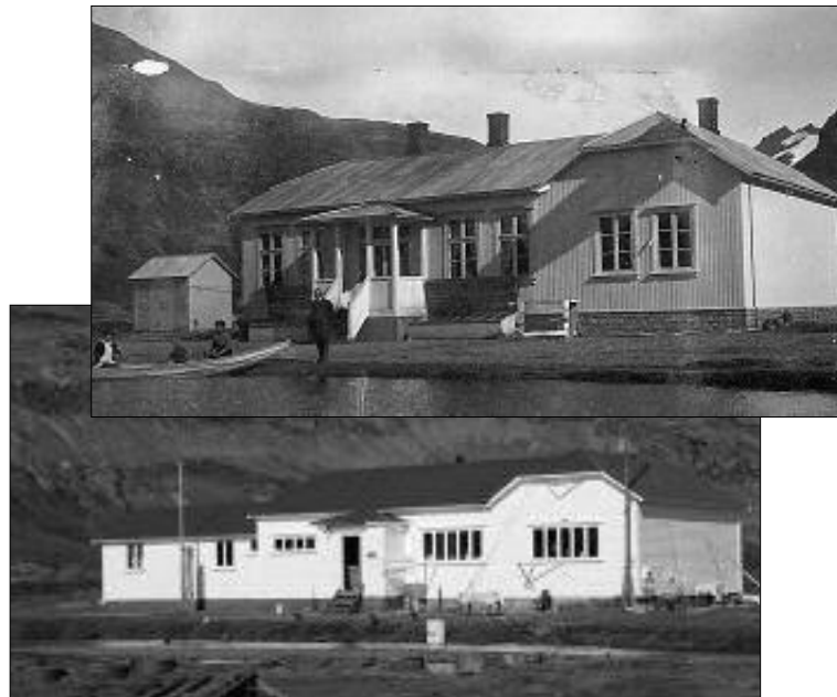
Husvik Villa: In the early days and after restoration..
