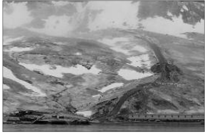
The temporary road to the dam.
