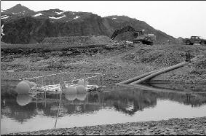
Siphon pipes emptying Gull Lake.
