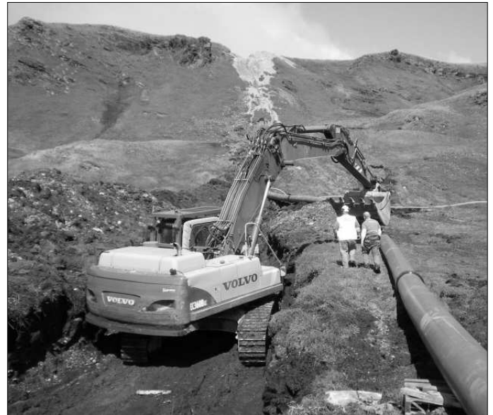
Laying the pipeline from Gull Lake.
