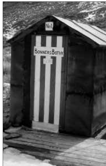
Bonner’s Bothy in October 1963 when it had become an emergency store. Its door had recently been painted for the first time and name boards attached.
