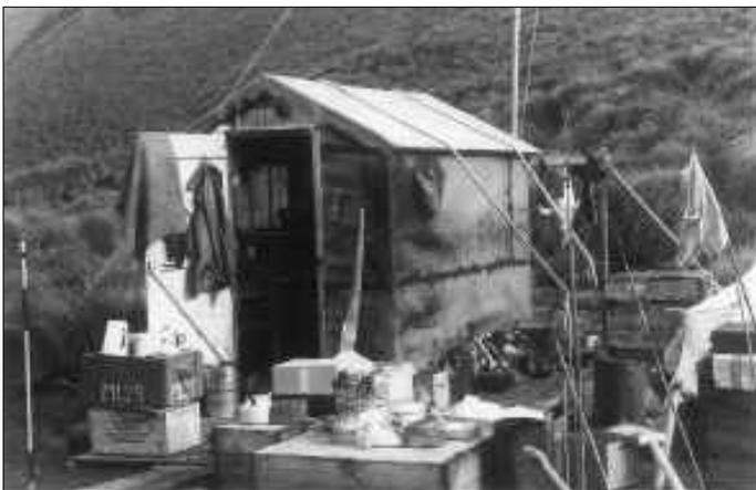
*In 1959 the walls were clad with roofing felt and the roof with sheet metal. It is clean-out day and the hut is surrounded by the contents of the hut stacked on decking.*
