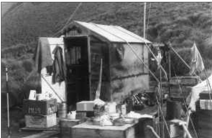
In 1959 the walls were clad with roofing felt and the roof with sheet metal. It is clean-out day and the hut is surrounded by the contents of the hut stacked on decking.
