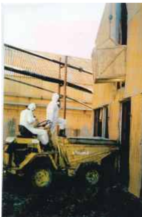
Removing a crate of asbestos.
