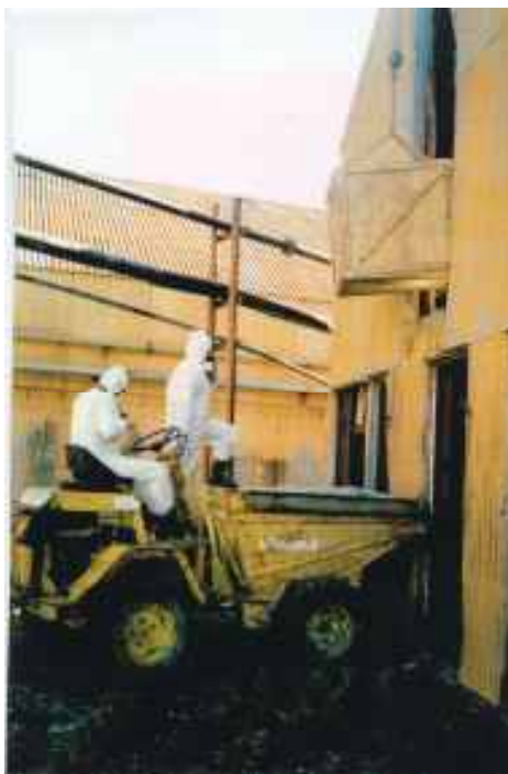
Removing a crate of asbestos.
