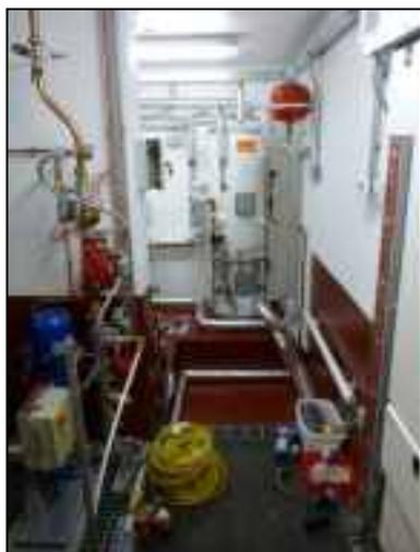
Part of the new boiler room. There is an electric boiler using power from the hydro-generator below Gull Lake and a diesel boiler as standby. The room also houses pumps for sewage and the fire sprinkler system.
