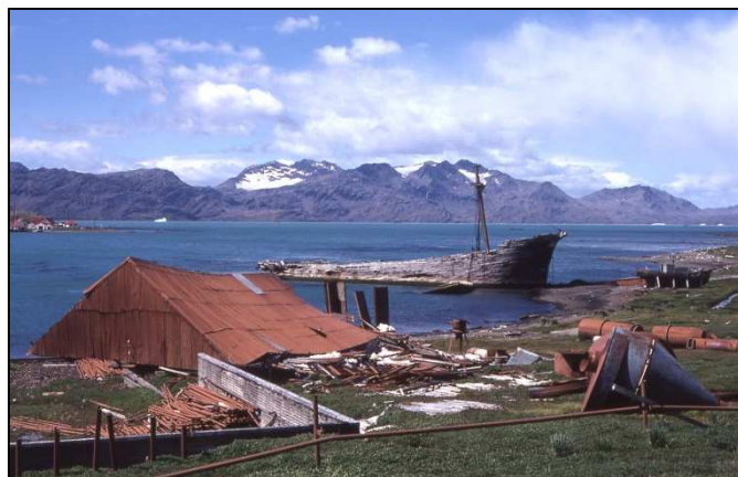
The collapsed Teatersalen on 1 February 1981, following the storm.
