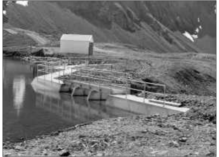
The rebuilt dam showing the spillway.
