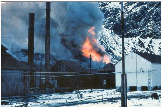
The fire appeared to have started in the electrical stores which also housed old diesel generators and was spreading rapidly. As well as the timber structure, there was oil, grease and other hydrocarbons in the building.
