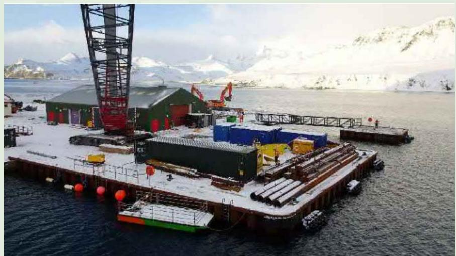
The dolphin, which extends the effective length of the wharf.
