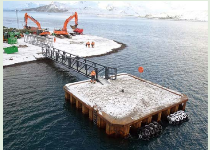
The dolphin, which extends the effective length of the wharf.
