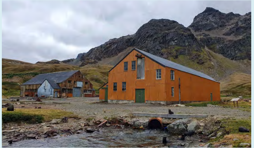
The main store at Grytviken with Engineers workshop to the left
