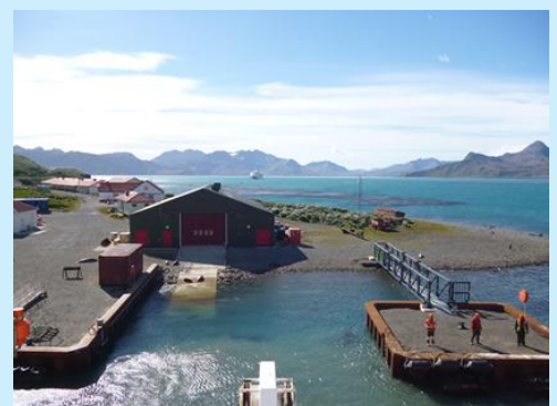
Arriving at KEP wharf – boatshed at the rear and the mooring dolphin to the right (Photo: A. Fox)
