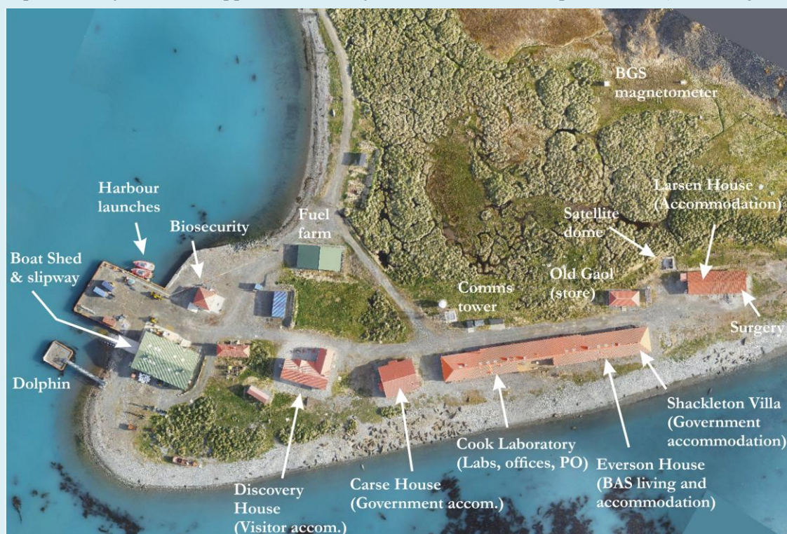
Drone image mosaic of the modern Research Station, with new priorities such as dedicated biosecurity building (Image: BAS/Nathan Fenney)
